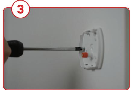
3 Secure the backplate against the surface, carefully filling in the two screw holes with the provided screws.
